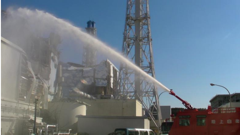
Fig.127 A fire engine responding to the accident in Unit 3 at the Fukushima-1 nuclear power plant, 15 March 2011. Author: Rikujojeitai Boueisho https://commons.wikimedia.org/wiki/File:23.3.22?_CRF:放水支援(3号機)※103隊撮影_東日本大震災における災害派遣活動_17.jpg
