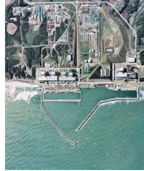
Fig.124. The Fukushima-1 nuclear power plant in 1975. Source: The Ministry of Land, Infrastructure, Transport and Tourism of Japan
