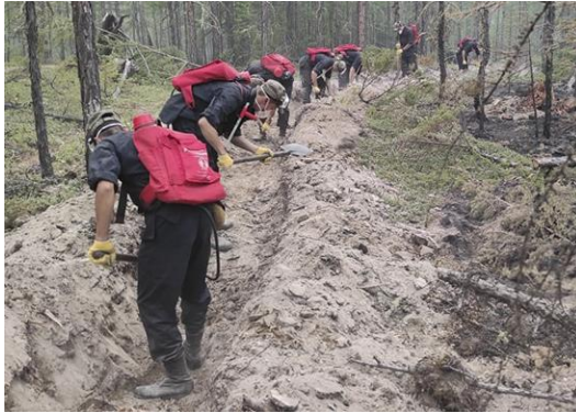
Fig. 120 Soldiers in Russia's Eastern Military District laying a mineralized strip in a forest to prevent the spread of fire. Yakutia, August 2021. Source: Russian Ministry of Defense
