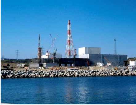
Fig.123 Construction of a protective dam at the Fukushima-1 nuclear power plant, 1970. Source: United States Department of Energy
